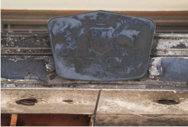
The fire-damaged front entrance of Old Parliament House following a protest.
