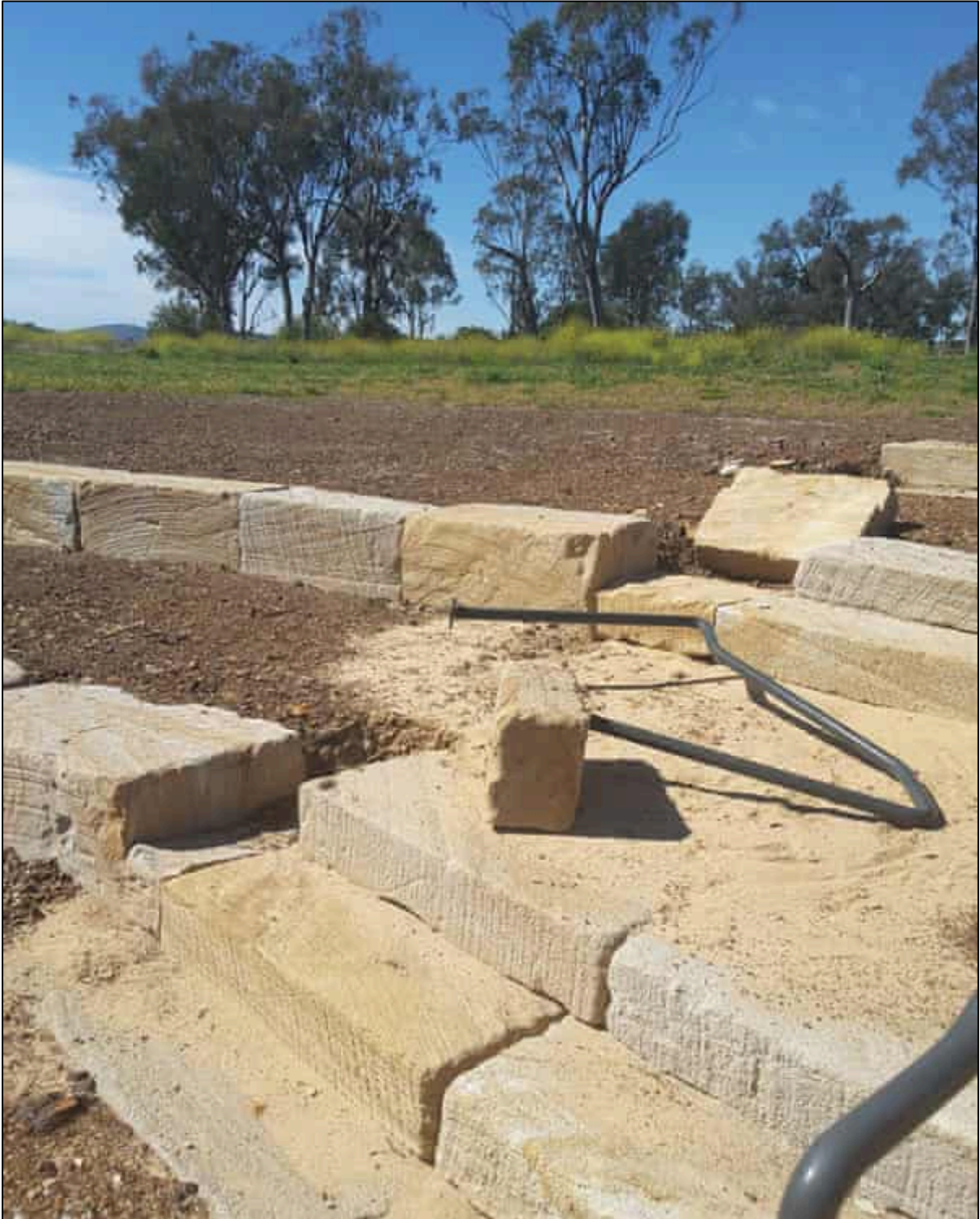
Damage to Myall Creek massacre memorial in NSW.
